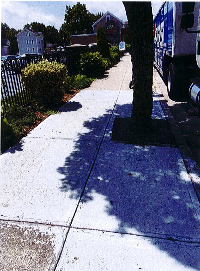
Sidewalk sections replaced, new pervious tree surround installed, and tree trunk wrapped with lighting
